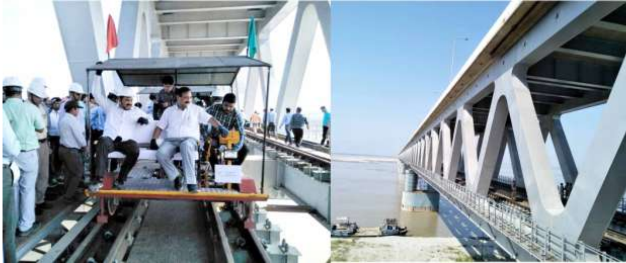
Shri S.K.Pathak,CRS, NF Circle and Shri S,N,Singh,CAO/Con-1 are seen conducting the inspection of Dhamalgaon to Tangani section of Bogibeel Bridge Project
